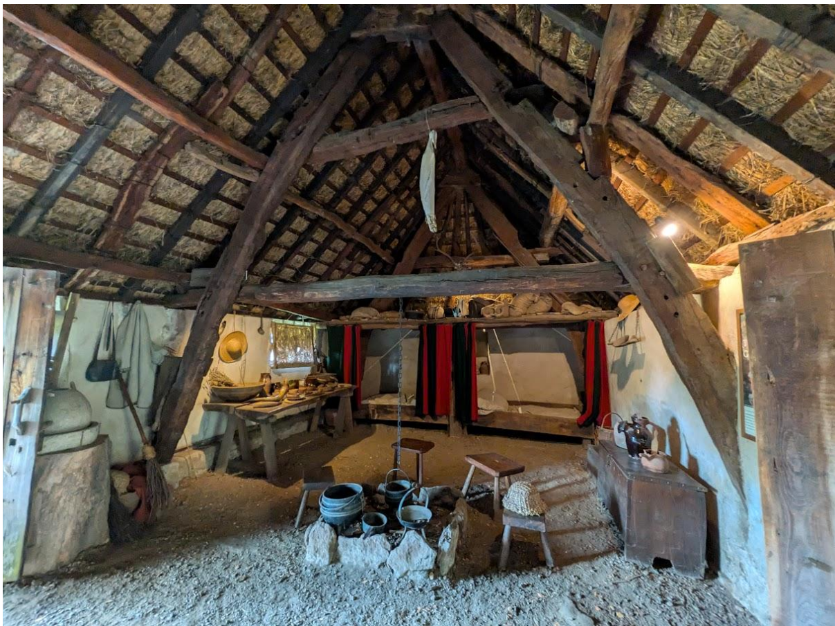
This reconstruction of a dwelling in the Ryedale Folk Museum (above) shows what the home of a prosperous peasant might look like in the North York Moors. Cruck-built
